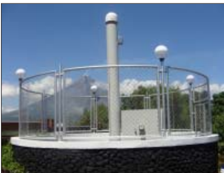
PLEG station in Legazpi City
