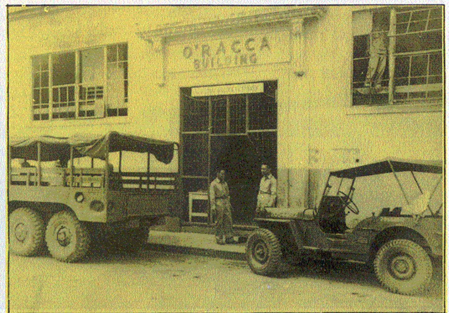
E. The old BCGS office in Binondo, Manila
